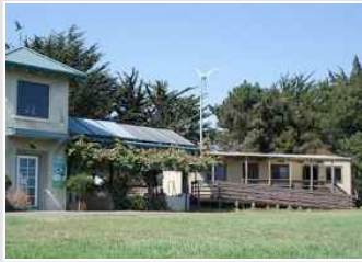
Photo Credit: Southwest Windpower
